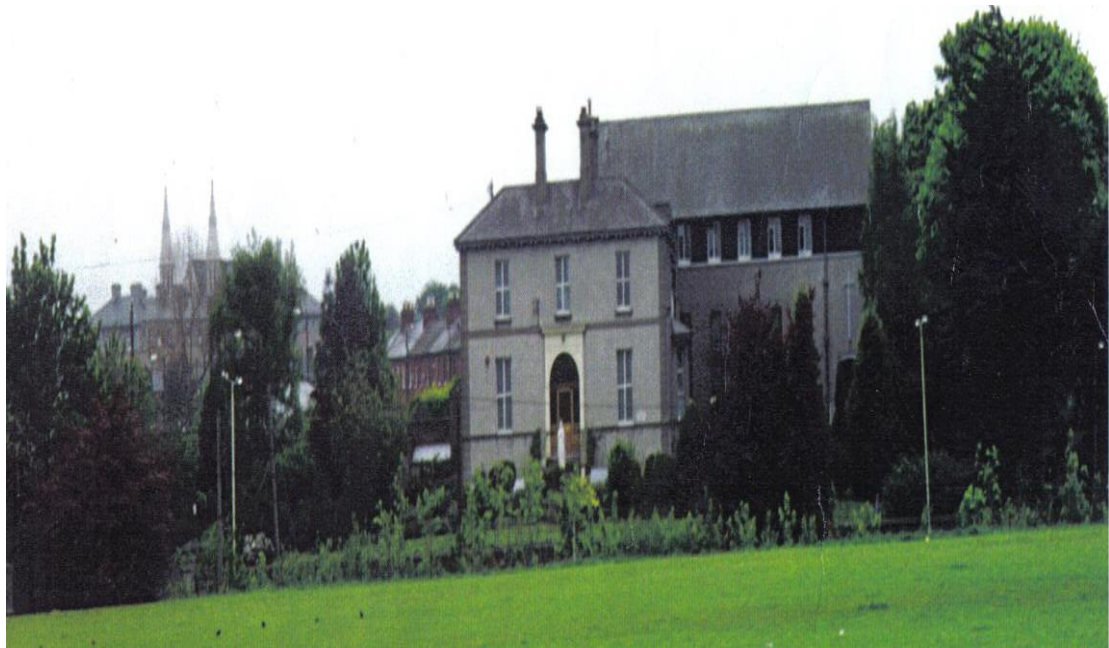
View of Sevenoaks Convent before the apartments showing the spires of the Oblates Church, Inchicore in the background
