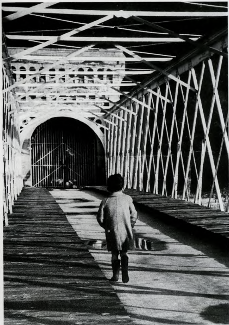
The bridge belonging to Lord Iveagh, which linked his lands on both sides of the river and carried the water pipe from a pump house to the top of the tower at Farmleigh. This attractive, latticed bridge now awaits restoration.
