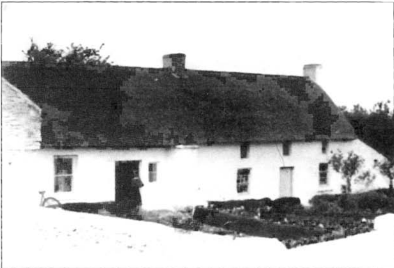
The Old Millhouse by the Camac at the Mill Bridge.
