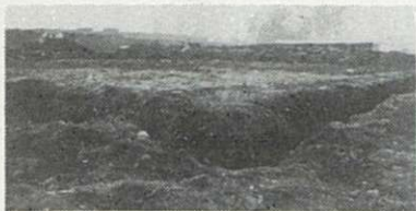
Digging the foundation
