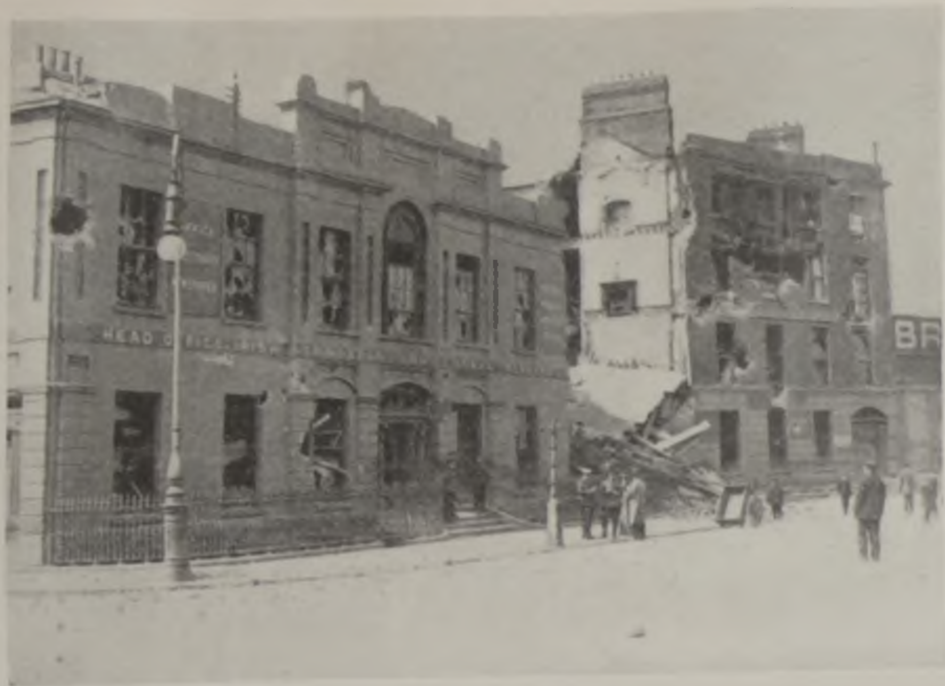
HEADQUARTERS OF THE IRISH REBELS. Liberty Hall, Dublin, was the chief stronghold of the insurgents in the Irish rebellion 1916. It was situated in Beresford Place, facing the Custom House
