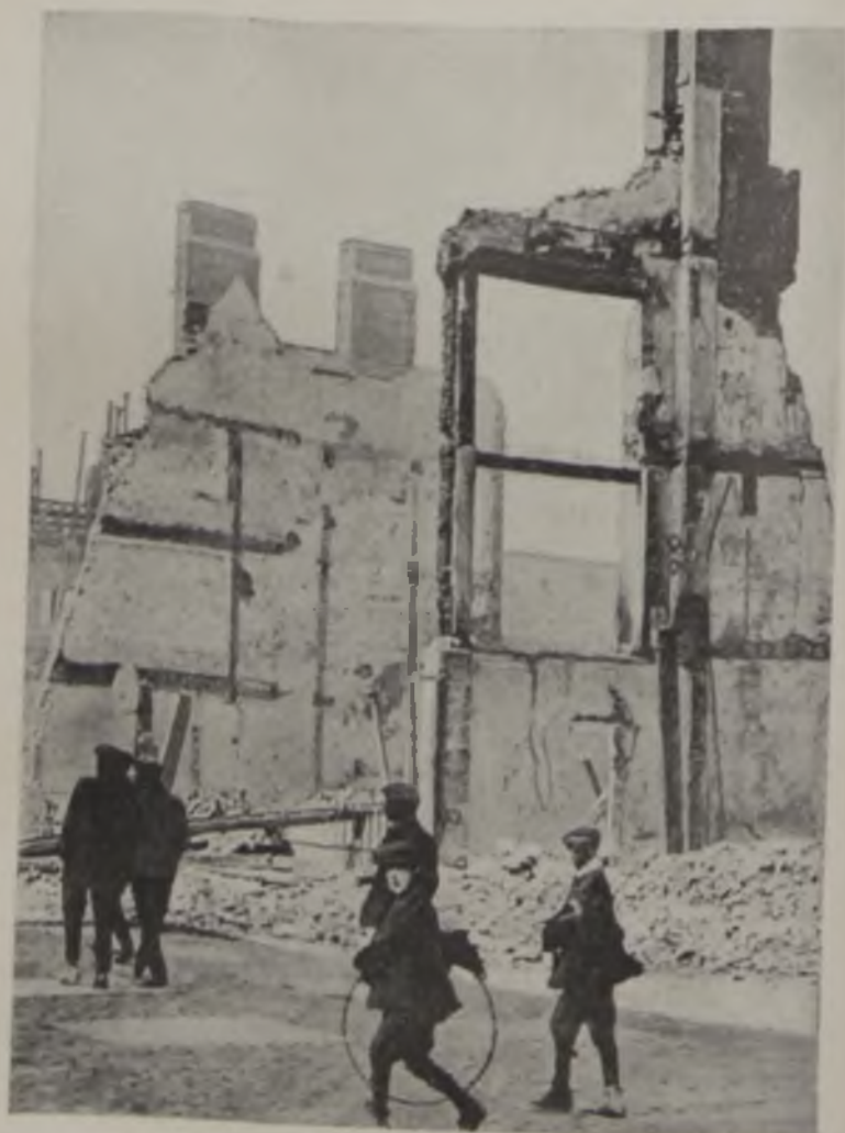
RUINS OF A REBEL STRONGHOLD. This photograph gives some idea of the damage caused in Dublin by the disturbances which broke out on April 24, 1916. When the rebels were driven from St. Stephen's Green by soldiers from the Curragh, they set fire to the buildings. There was serious destruction in the course of the fighting and the casualties numbered over 440 military and about 800 civilians. Outside Dublin the attempted risings reached no serious proportions.
