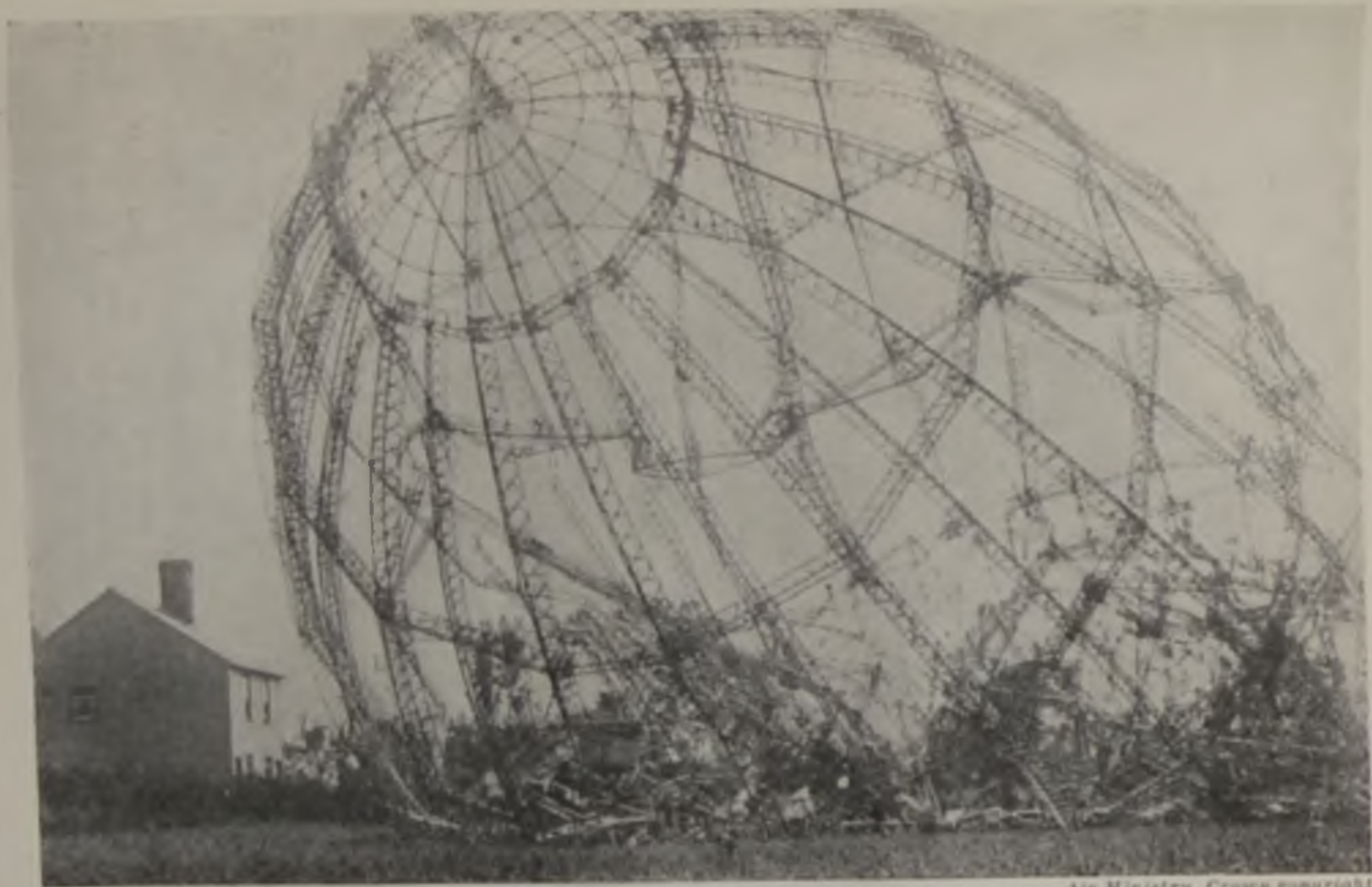
INGLORIOUS END OF A ZEPPELIN. One of the objects of the air raids over England was to intimidate the civil population. This Zeppelin, the L 33, is one that was forced down in a lonely part of Essex, through engine trouble and loss of gas, on the night of September 23, 1916.
