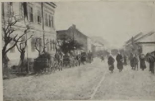
The main street of Kralievo in Central Serbia. The flourishing centre of an agricultural district, it suffered severely in the war. It fell to the Austro-Germans on November 5, 1915, and from here the Serbians began their retreat on Mitrovitza.
