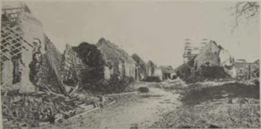
LOOS AFTER THE BATTLE. The ruins of the village of Loos, showing the famous "Tower Bridge," a pit-head structure, in the background. The battle, which was undertaken in September, 1915, with the object of recovering the French mining district around Lens, was preceded by a four days' methodic bombardment of the German positions. For the first time troops of Kitchener's New Army, raised in 1914, were employed.
