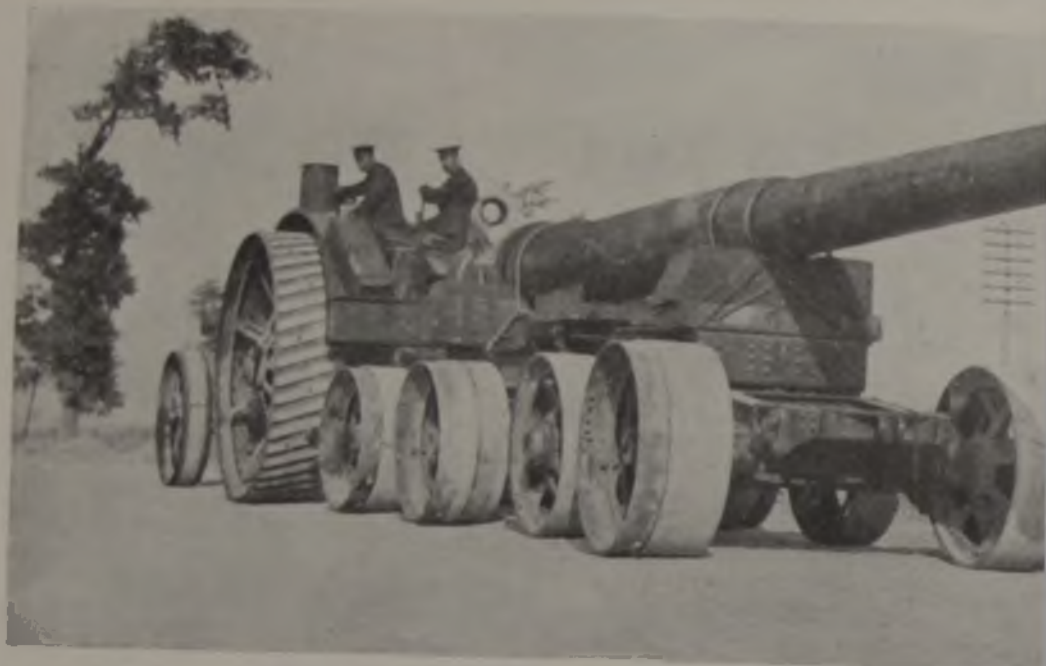
PONDEROUS INSTRUMENT OF DESTRUCTION. This is an epitome of the tactics that re-very end of 1917. A Royal Marine Artillery tractor is hauling the 15-ton barrel of a 7.5-in. long Swiftsure up to the forward area in July, in preparation for the 3rd battle of Ypres, which prov- the old tactical era.
