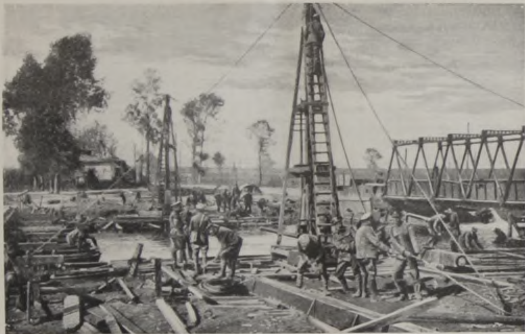
CANADIAN ENGINEERS BRIDGING THE CANAL DU NORD, NEAR CAMBRAI
