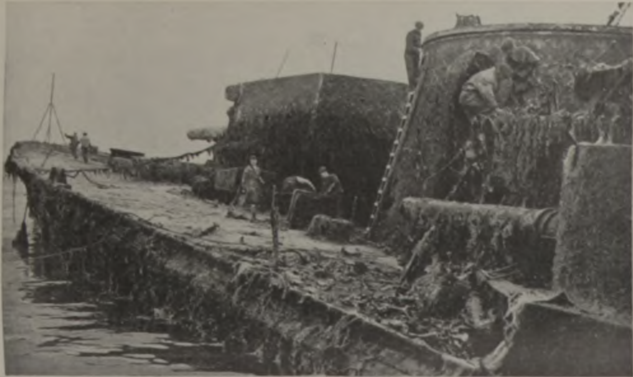
SALVING THE HINDENBURG. This remarkable photograph shows the 28,000-ton German battle cruiser, scuttled along with some fifty other interned vessels at Scapa Flow on June 21, 1919. Encrusted with seaweed and barnacles, it is in process of being raised from the bottom of the sea. The task of salvaging took four years, and finally the vessel was towed to Rosyth to be broken up in 1930.
