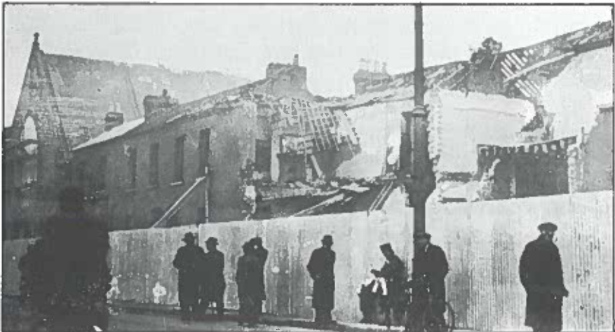
Bomb Damage, S.C.R.
