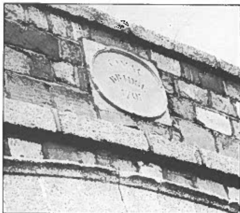
East Parapet of Dolphin's Barn Bridge
