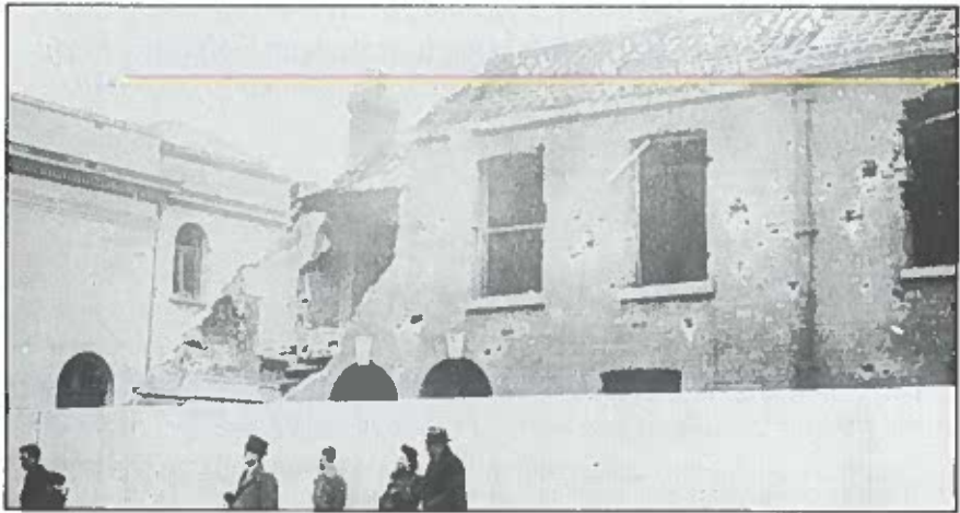
Bomb Damage, S.C.R.
