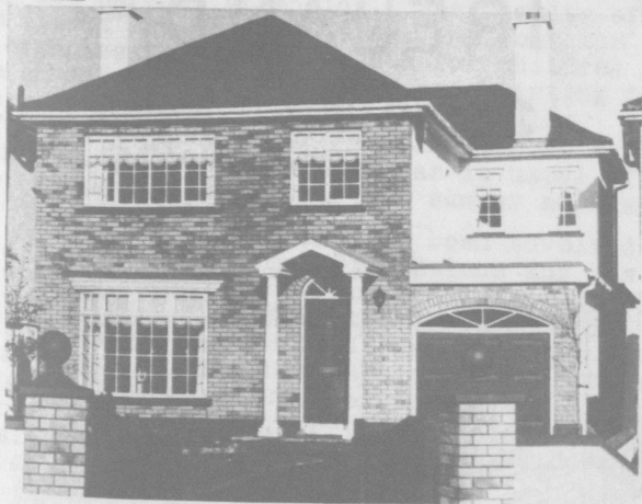
One of the new houses.
