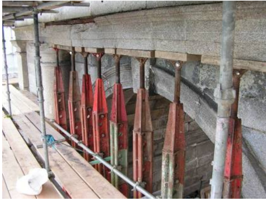
Shoring of the structurally unsound but historic and significant north-eastern entablature
