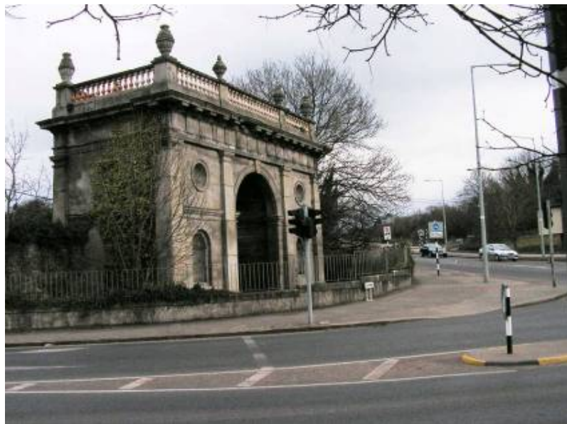
The Roman Arch viewed from the west, looking toward Braemor Road
