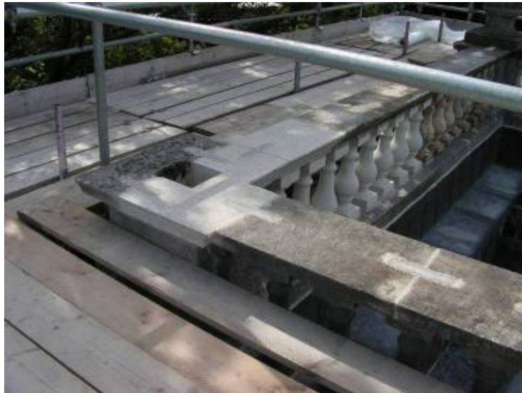
The south-eastern corner. New granite jointed with new stainless steel cramps.
