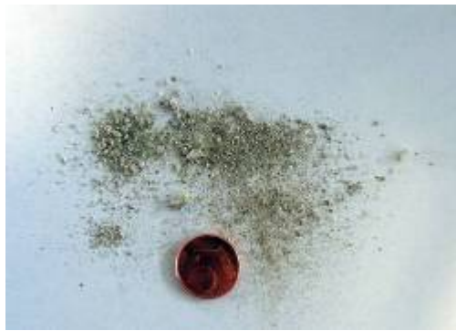
Mortar sample raked out from a joint in the south-eastern façade
