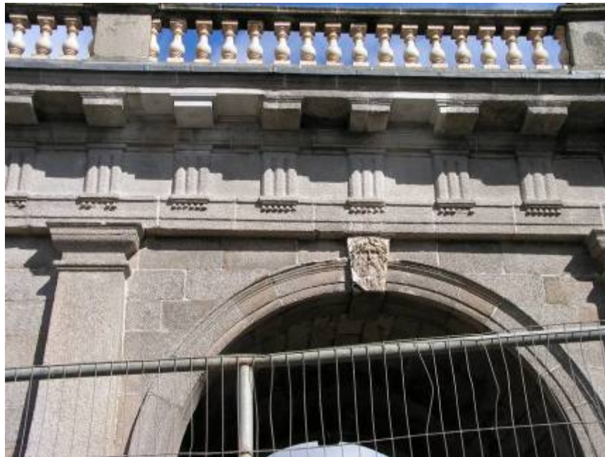
The south-western entablature: the completed repairs (photographed September 2010)
