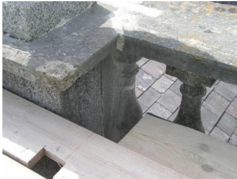
Existing limestone half-baluster on the south-eastern façade which was repaired
