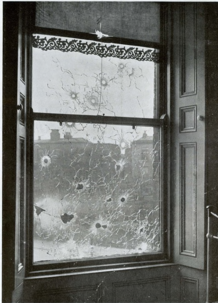
Bullet Pierced Bedroom Window in a Northumberland Road Mansion seized by the insurgents and used as a "fort."
