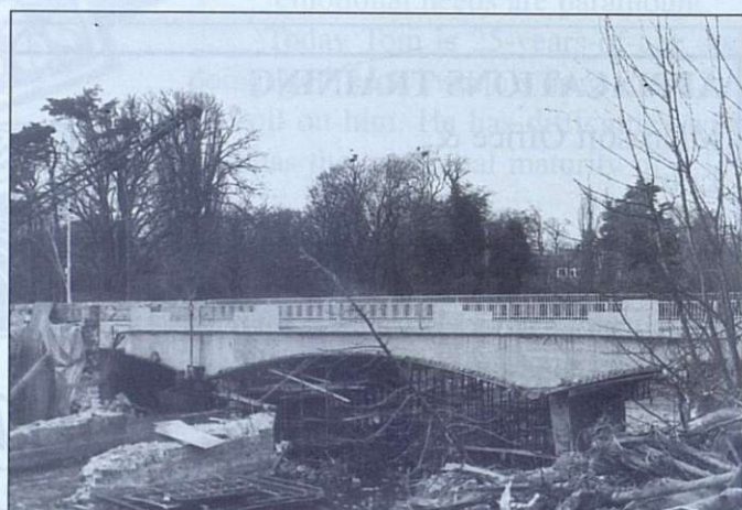
The Austin Clarke Bridge nearing completion and remains of old one.
